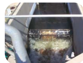
On discharge, the water treated has over 99% of any phosphorous removed.
